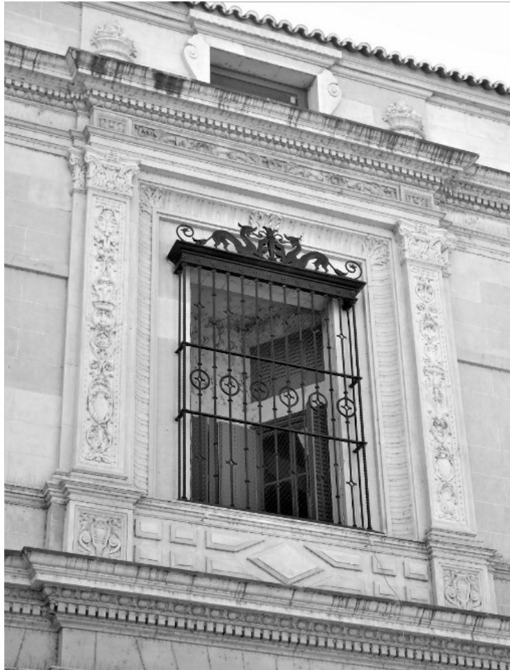
Fig. 08 – Detail of ornamentation and blacksmithing on the window of the west corner body. Source: architect Lelis Labuckas, 2019.
