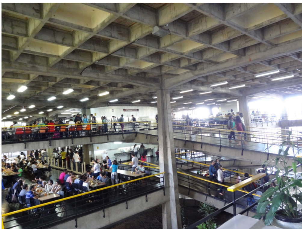
Fig. 9. Interior of the University Restaurant. Author: José Galbinski (1971). Photo: Eduardo P. Rossetti.
